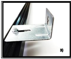
Set bottom jamb brackets approximately 100mm from the floor and for most 40mm thick doors set the track approximately 40mm from wall at the bottom and 70mm from wall at the flag bracket level. Adjust after second last panel is installed
