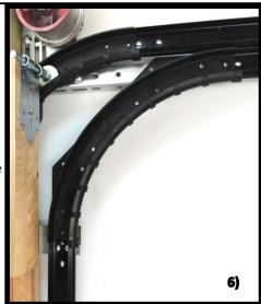
Low headroom set up shown is installed in 200mm headroom with vertical track cut to "ceiling height less 520mm". The main objective is to have the low headroom bracket flush or slightly higher than the panel. Bracket lower than the door may drive the door into the cable drum
